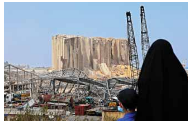
BEIRUT: A woman with her boy contemplate the damaged grain silos at the port of Beirut following a huge explosion that disfigured the Lebanese capital, on August 12, 2020. — AFP
