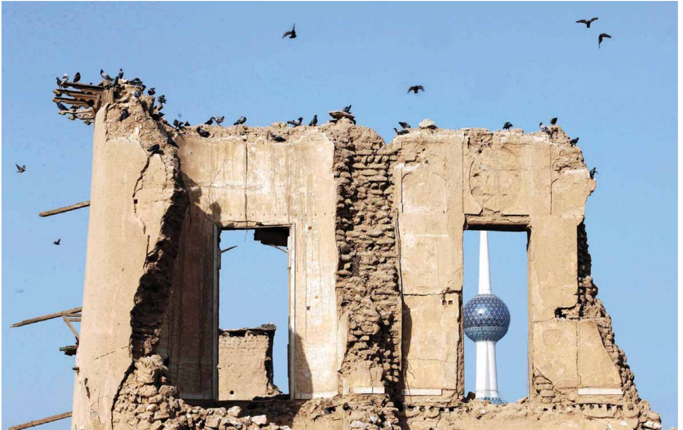
KUWAIT: Kuwait Towers seen through the window of the ruins of the Abdullah Al-Jaber Al-Sabah Castle in Kuwait City. The castle used to host a museum during the 1970s. — Photo by Joseph Shagra
